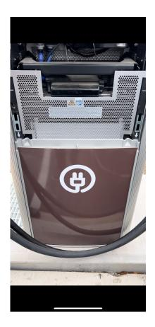
12. Align the guide tabs on the middle vent panel to the corresponding slots on the Express 250's frame. Ensure the lower sign is correctly captured as you carefully push the middle panel down until it is fully seated.
