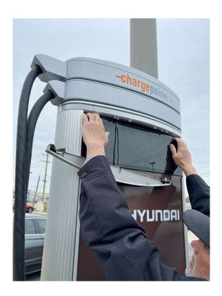
22. Ensure the gasket on each end of the new area light bar is properly seated around the plastic tab.
